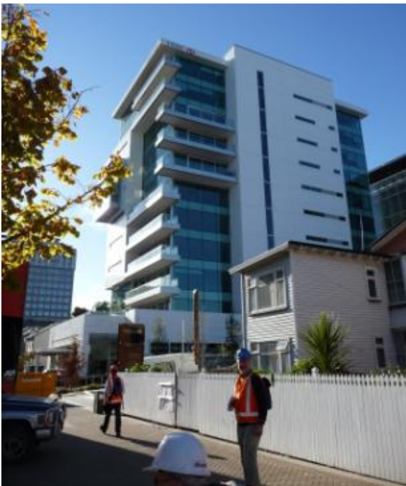
The 13 storey structural steel framed HSBC Tower on Worcester Blvd. was the first multi storey building re-occupied after the February 2011 Christchurch earthquake. The 2006 building designed to current steel construction guidance demonstrates that competitive technology exists to minimise potential earthquake damage
